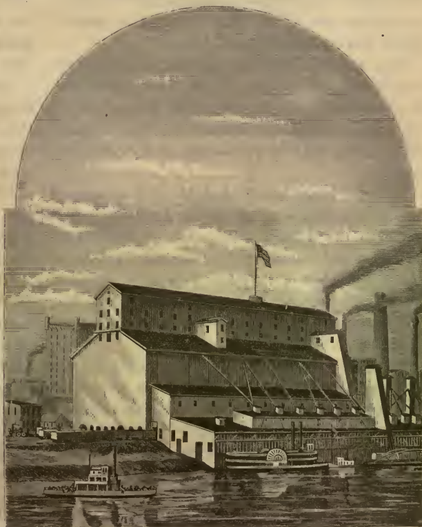
ST. LOUIS GRAIN ELEVATOR.
