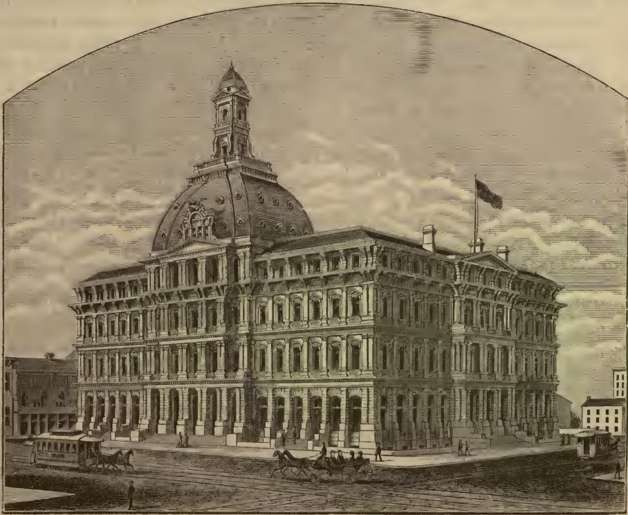
CUSTOM-HOUSE AND POST-OFFICE, Corner Eighth, Ninth, and Olive Streets.
